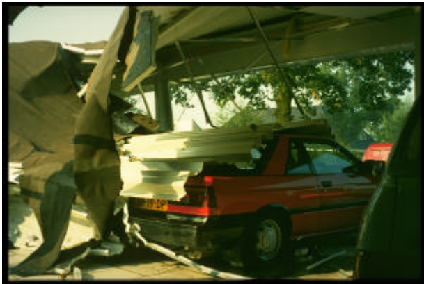
Photo 2 Detailed view of the roof opening. This is the place where the flash hit the roof.
