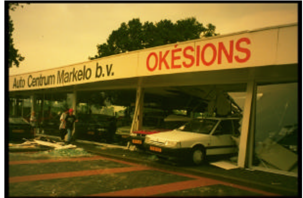
Photo 4 Front view of the building. Some cars were moved by the blast wave and ran through the pane of glass
