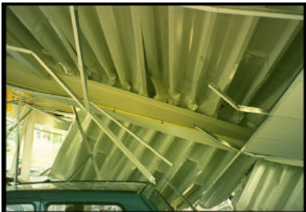
Photo 3 Smashed roof and twisted T-steel girder.
