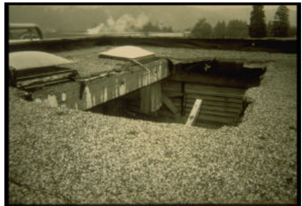
Photo 6 The roof of a paper factory in Austria after a lightning strike.
