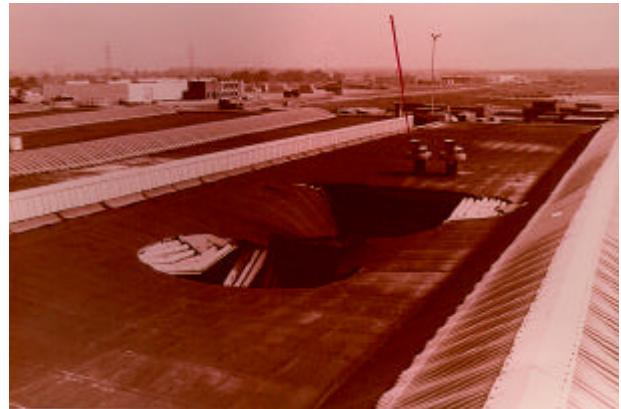
Photo 5 The roof of a Factory in Belgium after a lightning strike. The roof shows two big holes.
